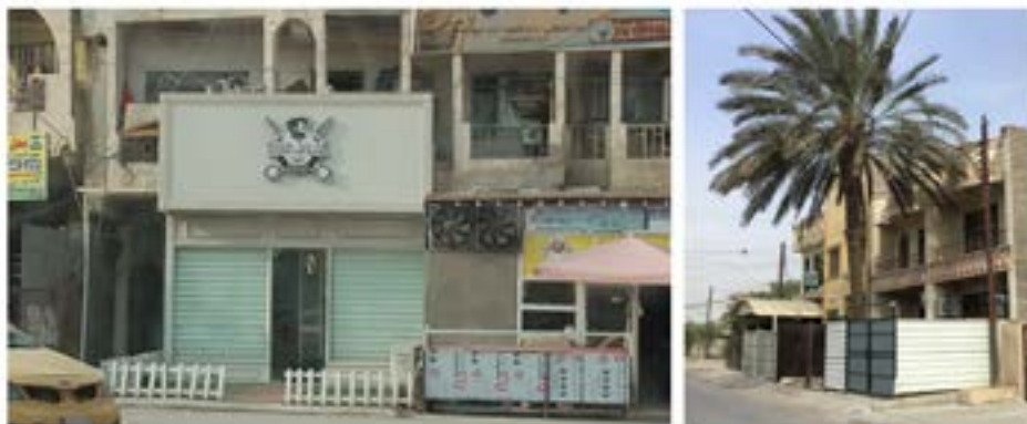
Figure 2. Images from Baghdad: The Construction Realm (author 2022)
